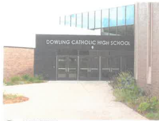
A1 MAIN ENTRANCE AND CHAPEL
