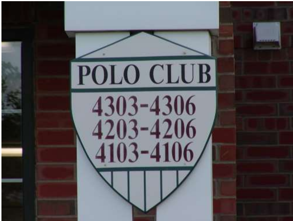
The first number indicates the building number (4000), the second number indicates the floor level (1=first floor, 2=second floor, etc.). The following numbers indicate the apartment number. Minimum 3 inch high, ½ inch stroke.
